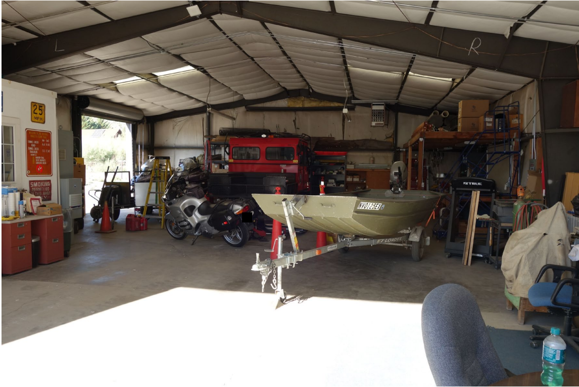
Marlette Lake Office / Storage Building – FCA Building #2488 Description: Interior of the Building.
