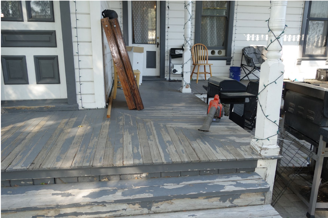
Lakeview House – FCA Building #2484 Description: Deck Refinish Needed.
