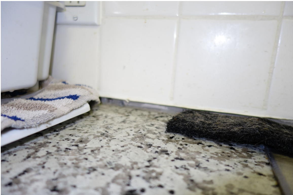
Lakeview House – FCA Building #2484 Description: Kitchen Backsplash Replacement Needed.
