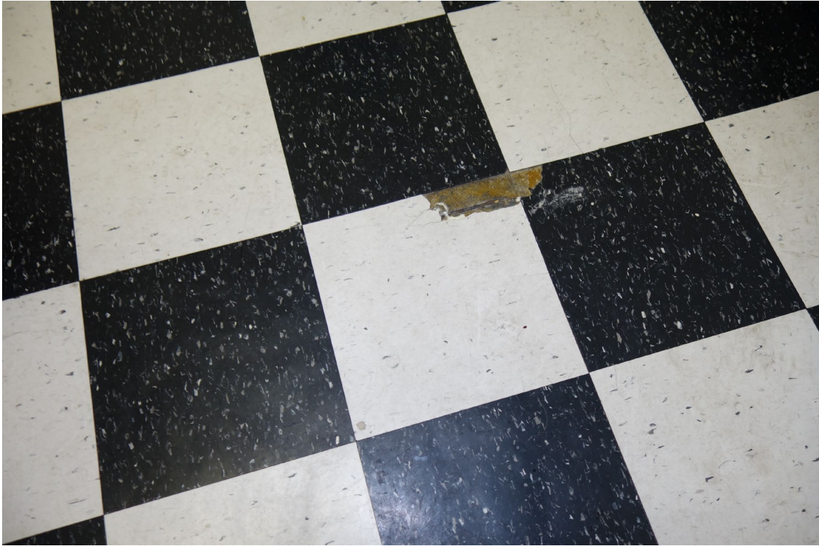
Lakeview House – FCA Building #2484 Description: Kitchen Flooring Replacement Needed.
