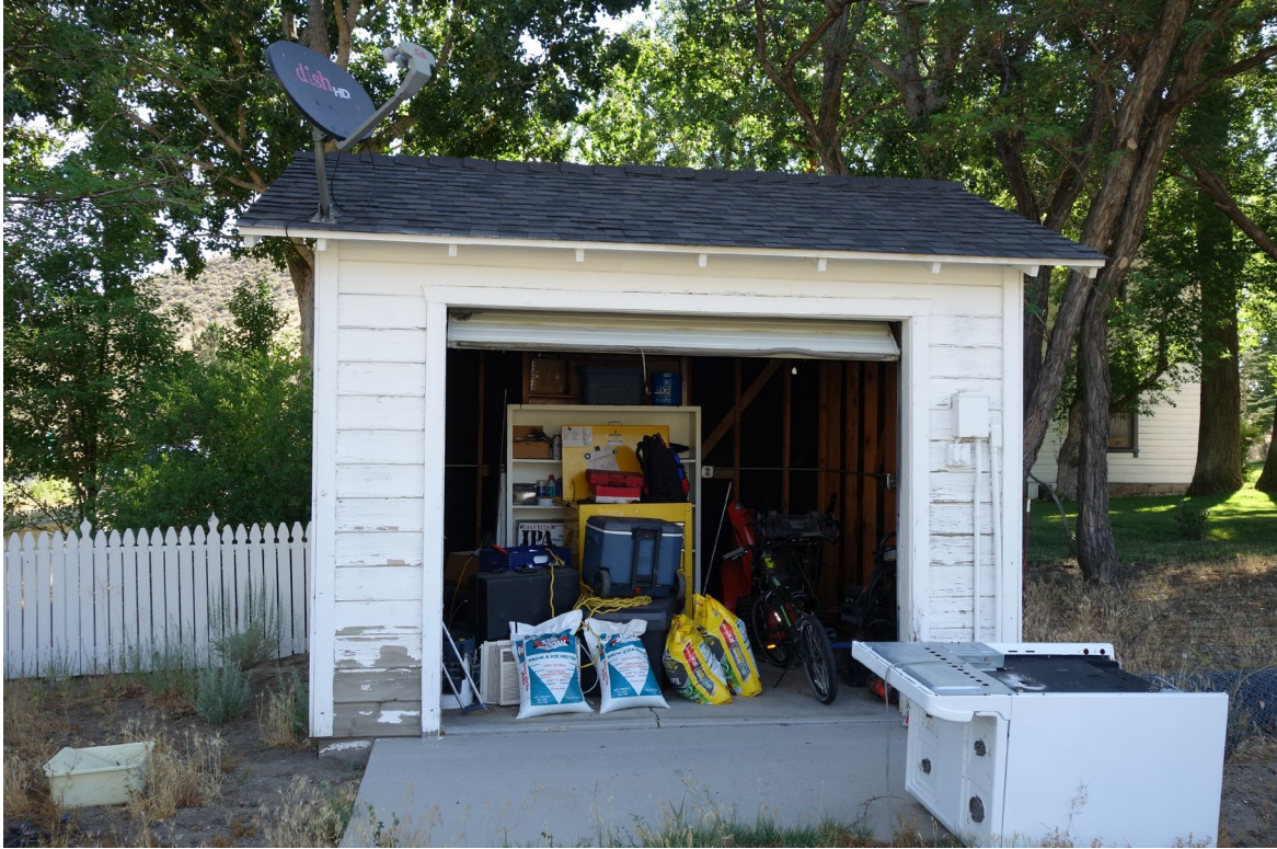
Water Master House Shed – FCA Building #2498 Description: Exterior of the Building.
