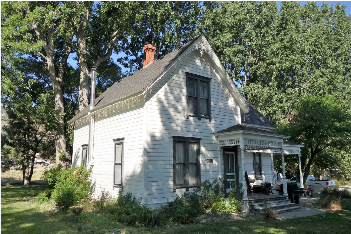
Lakeview House – FCA Building #2484 Description: Exterior of the House.
