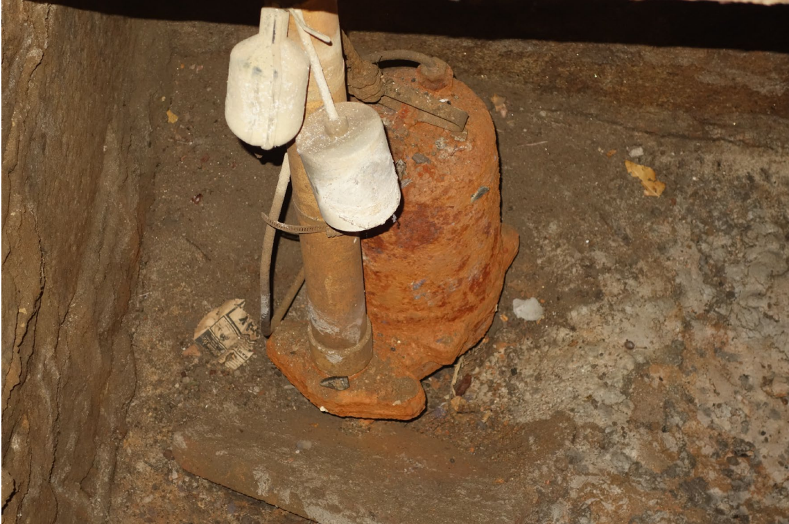
Lakeview House – FCA Building #2484 Description: Sump Pump Replacement Needed.
