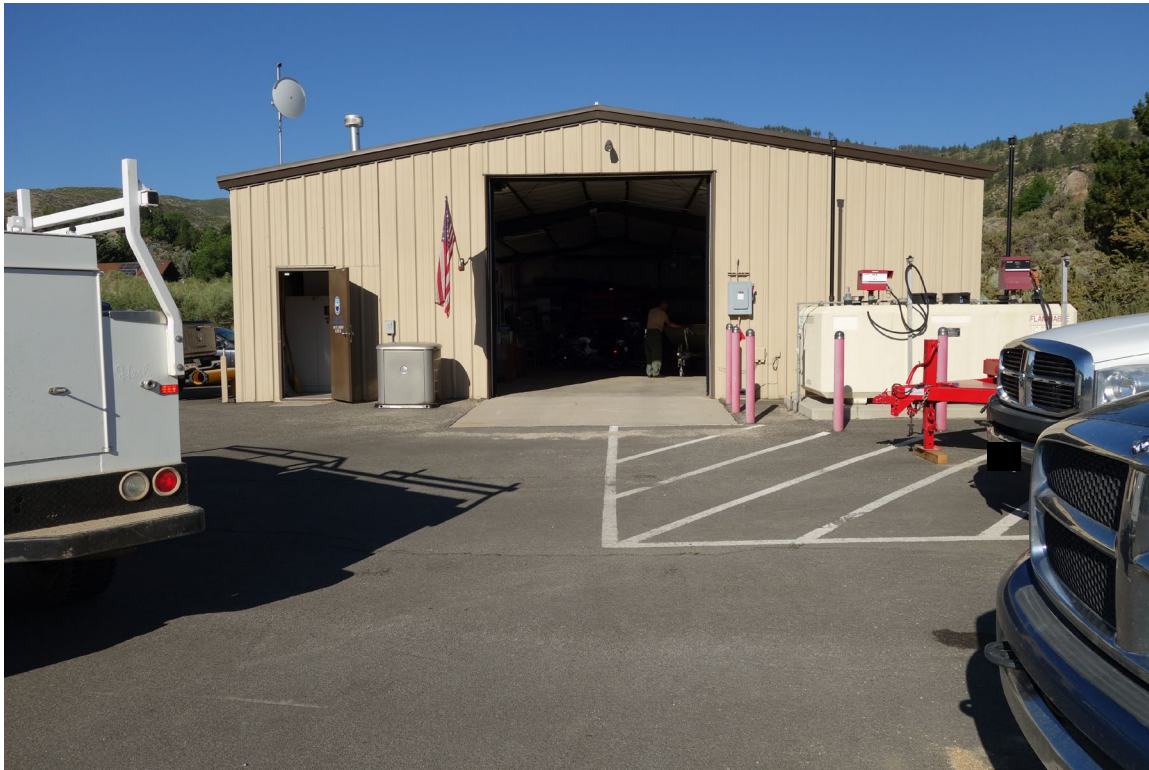
Marlette Lake Office / Storage Building – FCA Building #2488 Description: Exterior of the Building.
