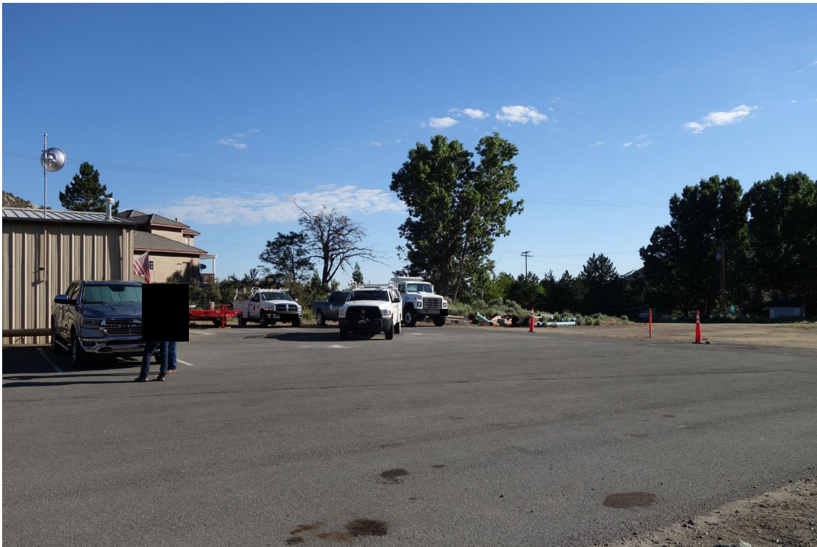
Marlette Lake Water System Office Site – FCA Site #9899 Description: View of Site Lacking Site Lighting.
